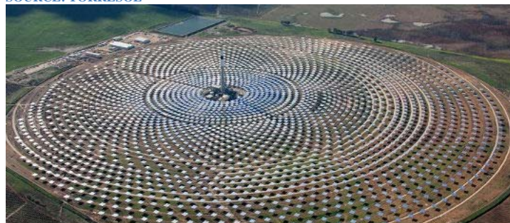
Torresol Gemasolar Solar Thermal Power Tower, Spain SOURCE: TORRESOL
